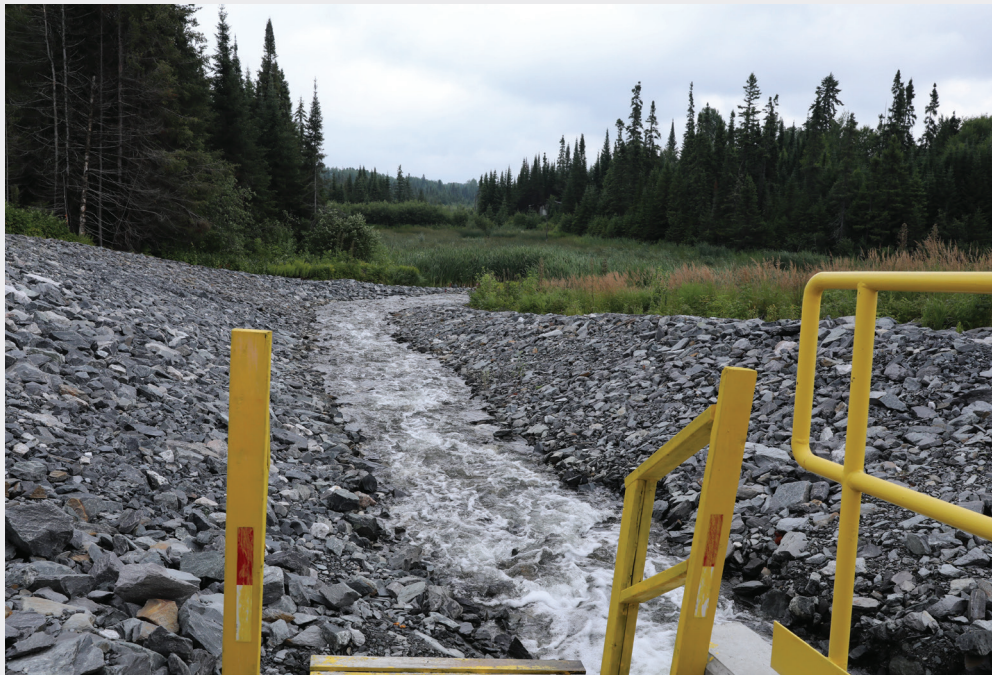
To avoid immediately killing wildlife, water from the mine must be treated to raise its pH from 2–3 to 5–6. Here, treated water is released into the boreal forest. PHOTO: ORIT HALPERN.
